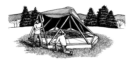
Without a third person position the base of the side support poles so they rest against each other allowing one person to reach down and bolt the base eyebolts together.
